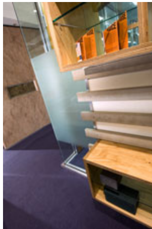
Detailed view of recycled plastic slats featured in Zero Waste SA's reception area
