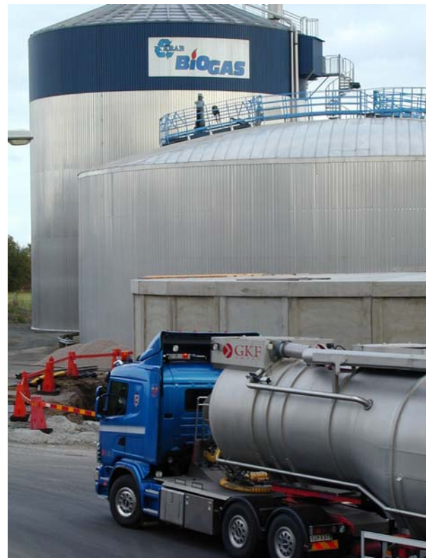
Figure 6: Anaerobic Digester, Kristianstad, Sweden
