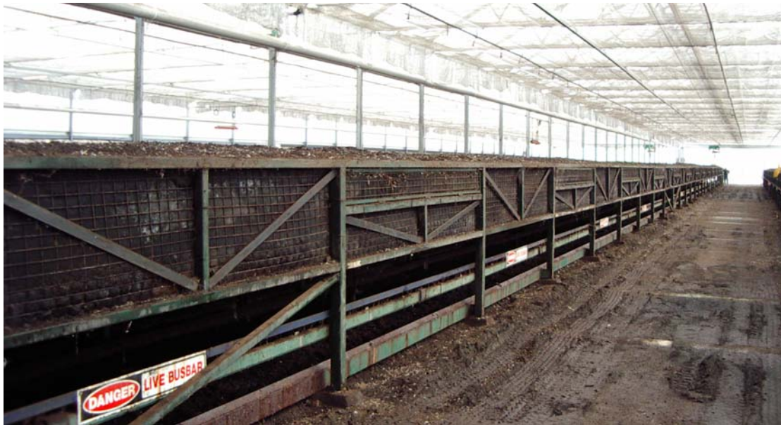
Figure 5: Tryton Vermiculture Facility, Lismore, NSW
